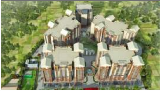
BCC ESTATE 3 BHK APARTMENTS Gomti Nagar, Lucknow
